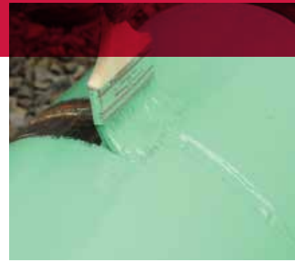
Applying pipe coating to weld seams.
